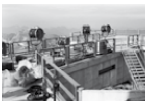
Below: The ice tunnel is finished, the heliport prepared for shooting.
